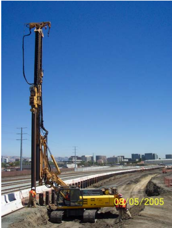
H-Pile installation alongside an active railway.
